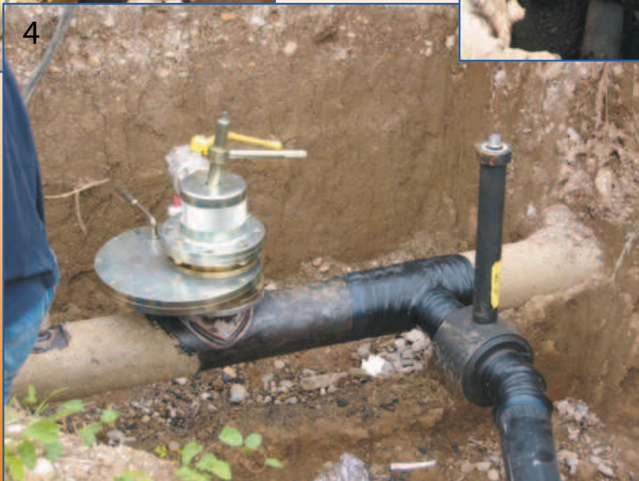
Foto 4 Tamponatrice DN 6" Plugging machine DN 6"
